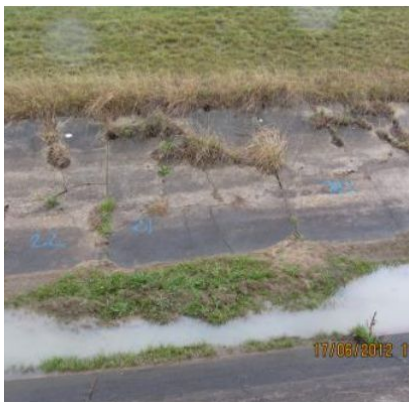
Figure 1. Open concrete water supply channel BEFORE remediation with Geofabric and Elaston-W80 polyurea
