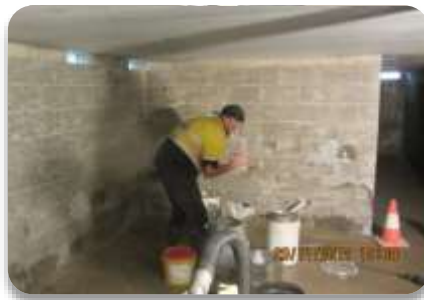
Figure 2 Typical below floor tanking preparation
