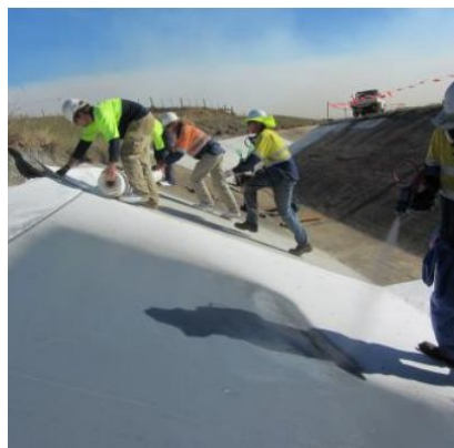
Figure 2. Open concrete water supply channel DURING remediation with Geofabric and Elaston-W80 polyurea
