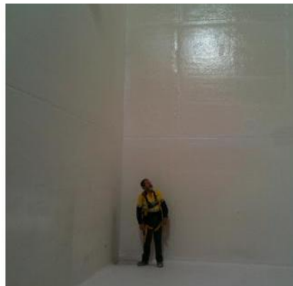
Figure 2. Water treatment plant concrete holding tank lined with Tufflon-P90.
