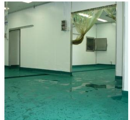
Figure 3. Seafood processing factory floor coated with non-slip green Tufflon-P90.
